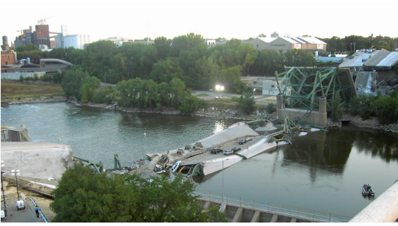
Figure 1.1: During the evening rush hour on August 1, 2007 the I-35W Mississippi River bridge collapsed killing 13 persons. Federal inspection had ranked the bridge structurally deficient, like about 70,000 other bridges in the U.S.
